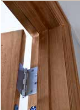
Double Rabbet, 90-Minute, with Clips (clip removed and clips attached)
